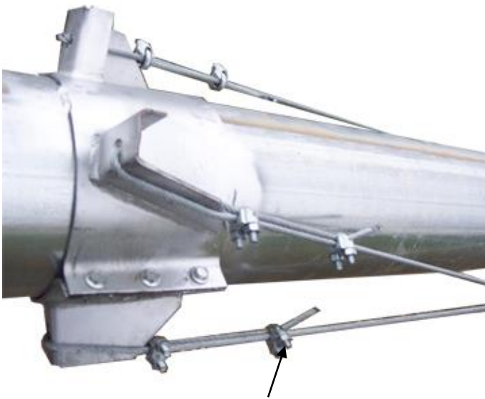
Cable clamp must be fastened with looped end over free end of cable otherwise slipping will occur.
