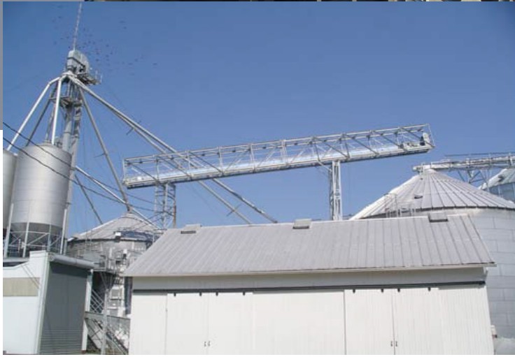
Cantilever Catwalks No Roof Loads
