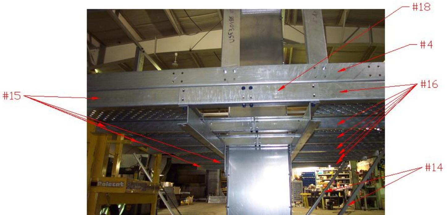
7. To make it easier to install the toe boards (4" X 2" angles) and floor panels, lay them out on the ground as shown in the picture below. (For both types)
