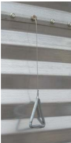
Figure 60 Sweep Stop Cable
